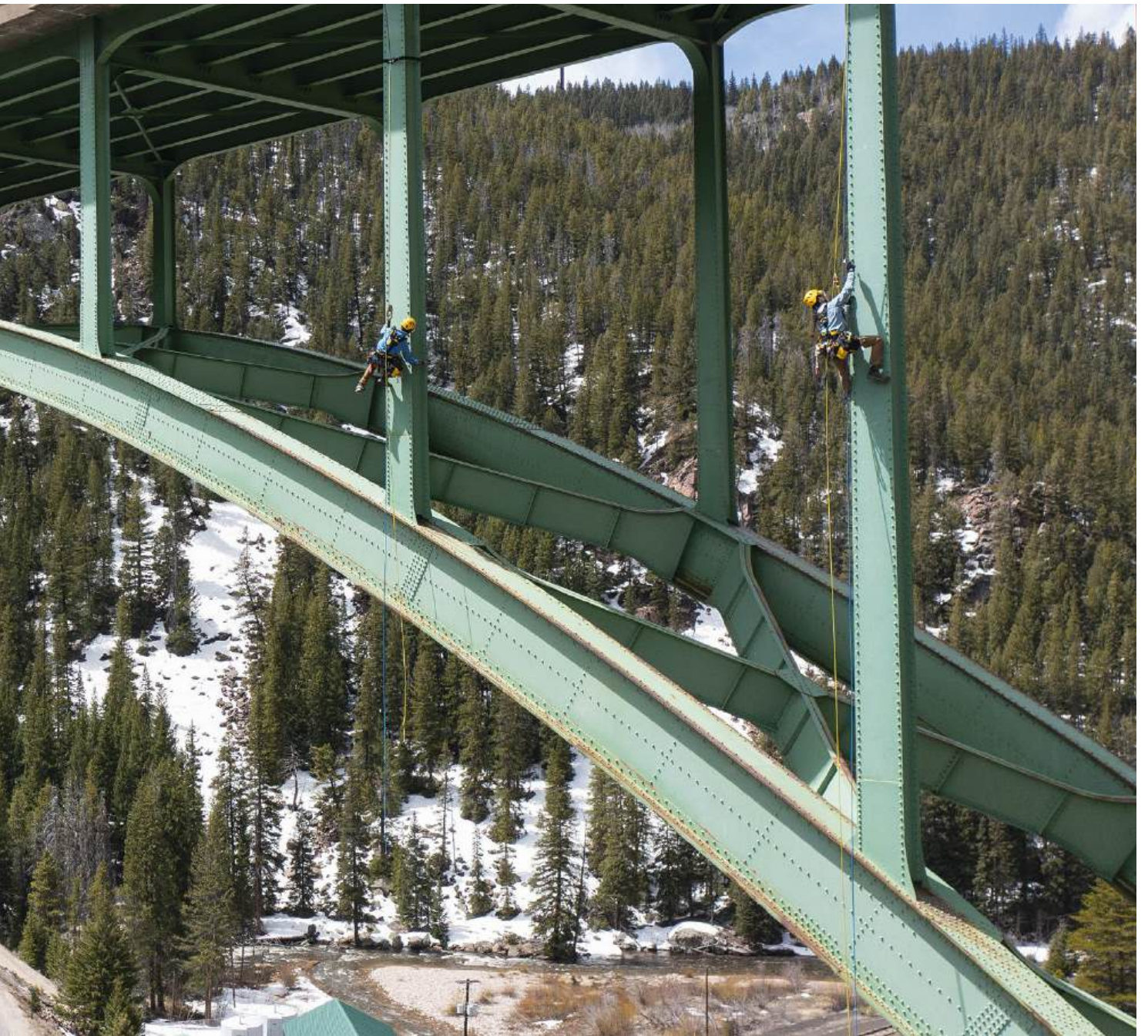
Bridge inspection, Red Cliff Bridge, Colorado, USA © 2024 - Petzl Distribution - Vuedici.org - Lafouche
