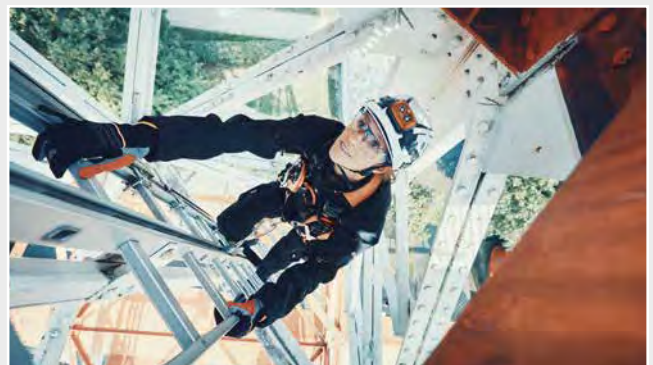
SPEED ATTACH on SÖLL GlideLock rail (Honeywell)
